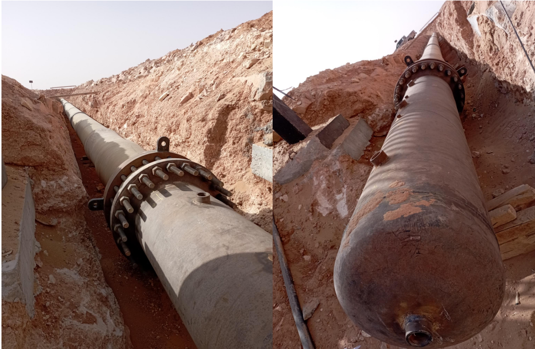
Figure VI.16: Test hydrostatique
