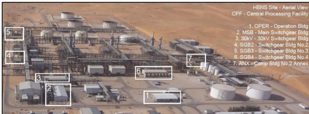
Figure 4.2: Aerial Overview of HBNS Site's CPF.
