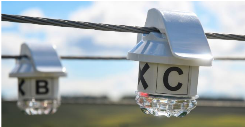
Figure 1. Overhead line fault passage indicators [3]
