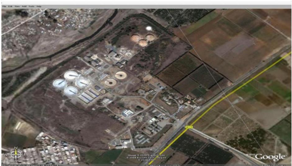
Figure 1.1: Aerial View of the Algiers Refinery.
