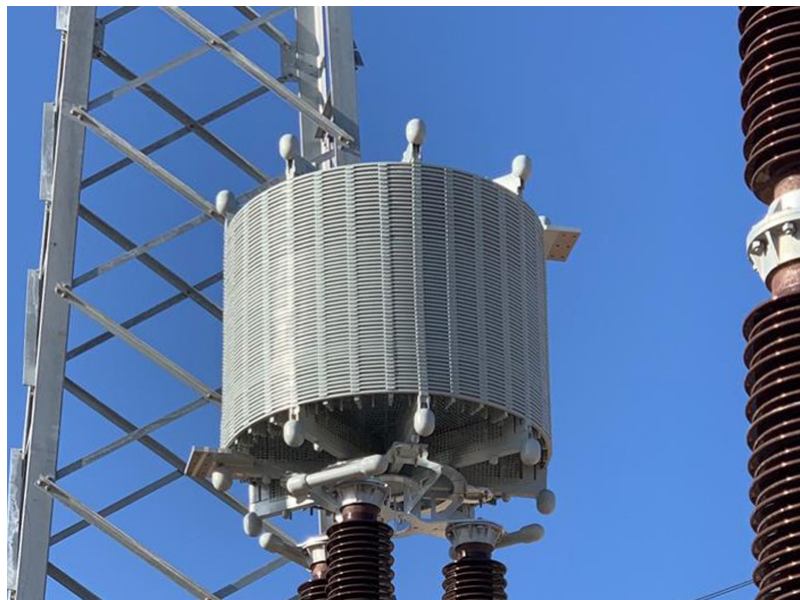
Figure 1.16: Line trap.
