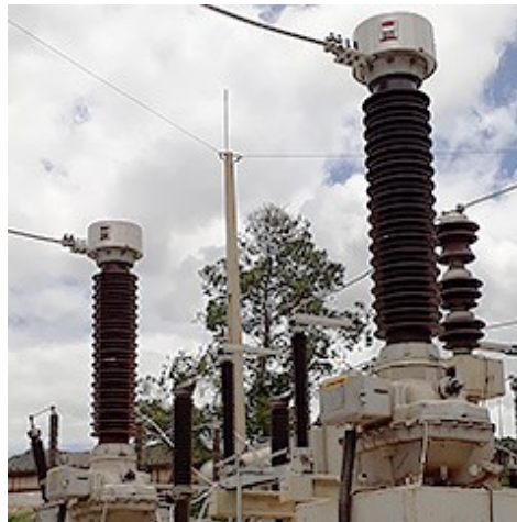
Figure 1.12: Voltage transformer.
