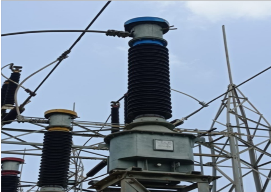
Figure 1.10: Current transformer.
