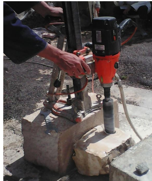
Figure III.2: carottage de pierre
