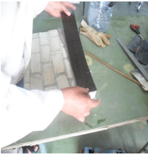
Figure III.34: pose de tissu de carbone
