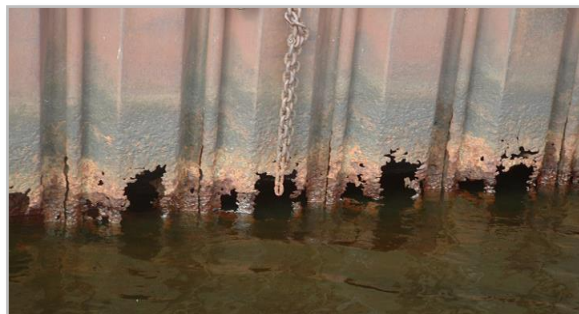
Figure III.2. MIC des pilotis, ([A], 2020)
