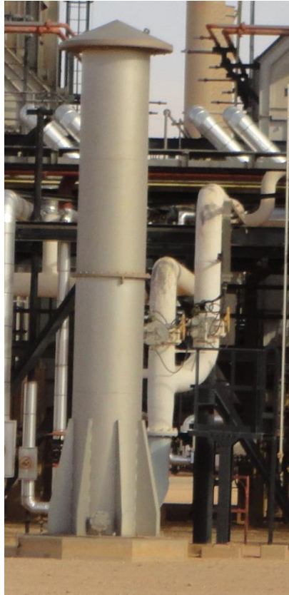
Figure II.9: Soufflante K102.
