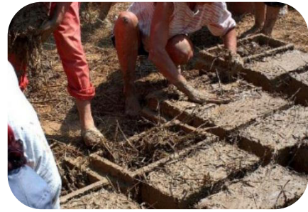
Figure. I.3 making bricks with straw and mud [11]
