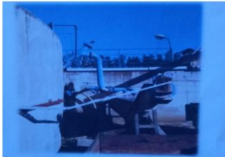
Figure.I.13: Ejector aeration unit (Air lift).
