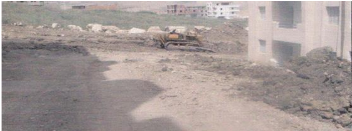
Figure VI-5: Reprofilage de la pente
