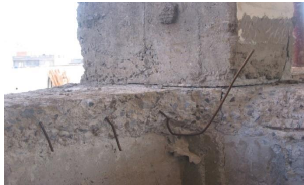
Figure IV-11: Fissures des longrines
