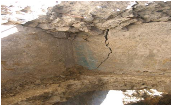
Figure IV-11: Fissures des longrines
