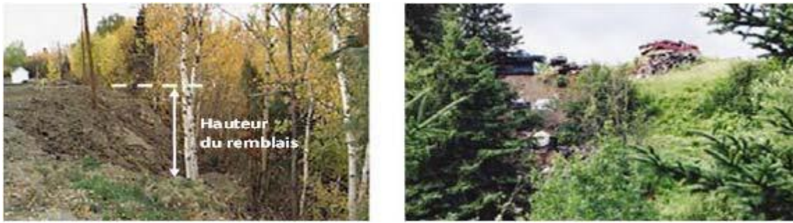
Figure I-18: Surcharge au sommet de talus
