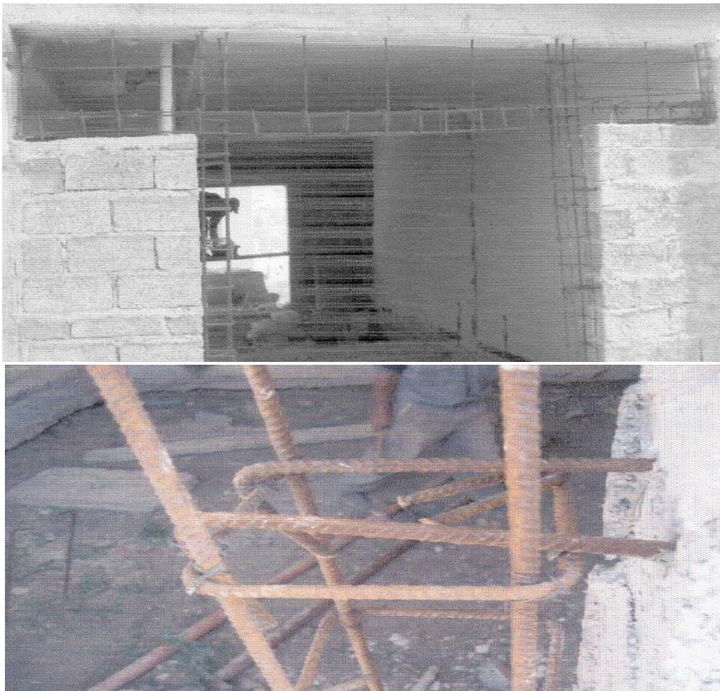
Figure VI-8: Chemisage des poteaux
