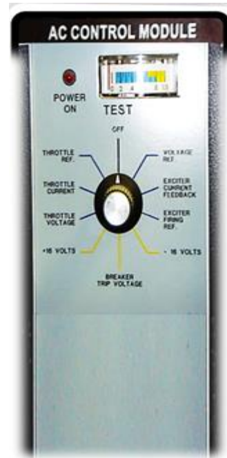
Figure 3.3 : Module AC control
