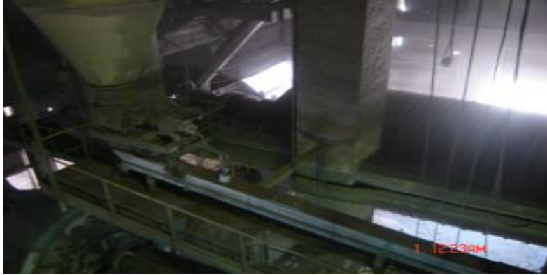
Figure I. 13 : Atelier Broyage ciment
