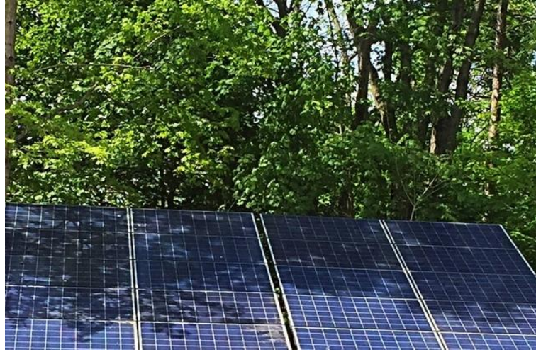
Figure 2.8 PV panels under shading.
